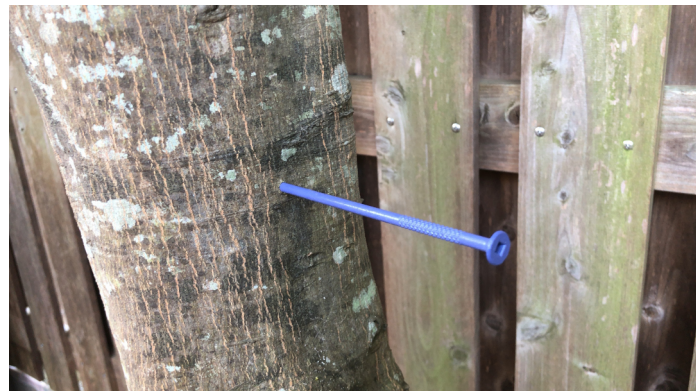
7. Insert until the screw part is hidden
