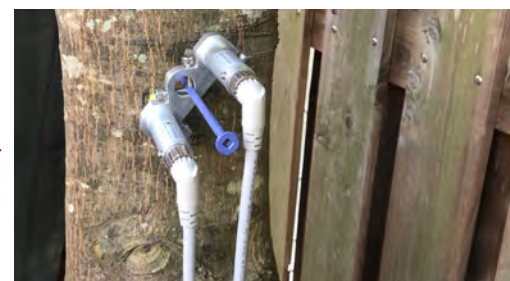
15. Make sure that cable is straight down toward ground.
